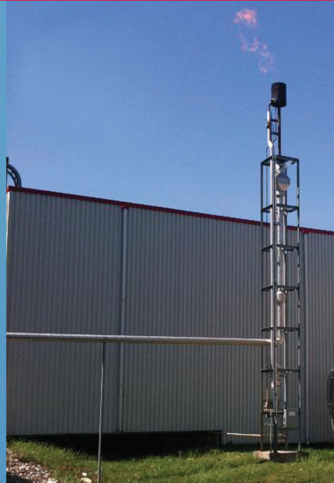
Biogas Flare that produces 2.5 MMBtu/hr of energy that is not being utilized and the associated testing equipment to track methane concentration
